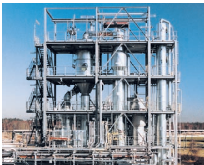
Two-effect falling film forced circulation evaporation plant in counter-current arrangement, with downstream distillative cleaning of the vapour condensate. Evaporation rate: 9,000 kg/h with a concentration to 65 % TS (dry substance)
