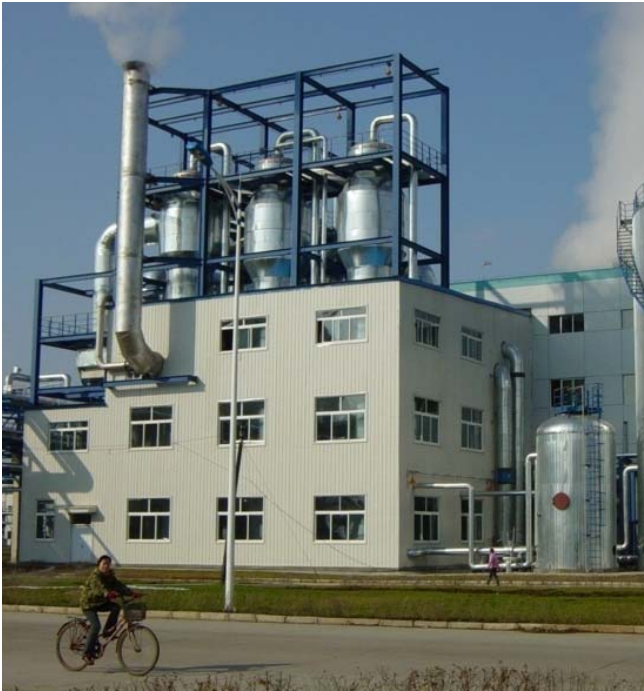
Fig. 7: 5-effect falling film and forced circulation evaporator, heated by dryer exhaust vapour, concentrating 140 tonnes/hr of stillage from 6.6 % to 35 % TS, arrangement C
