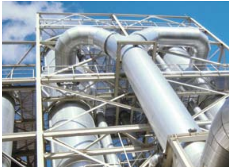
EVAPORATION PLANT for the concentration of waste waters and effluents from wheat starch production heated by means of a mechanical vapour recompressor. Evaporation rate: 30,000 kg/h
